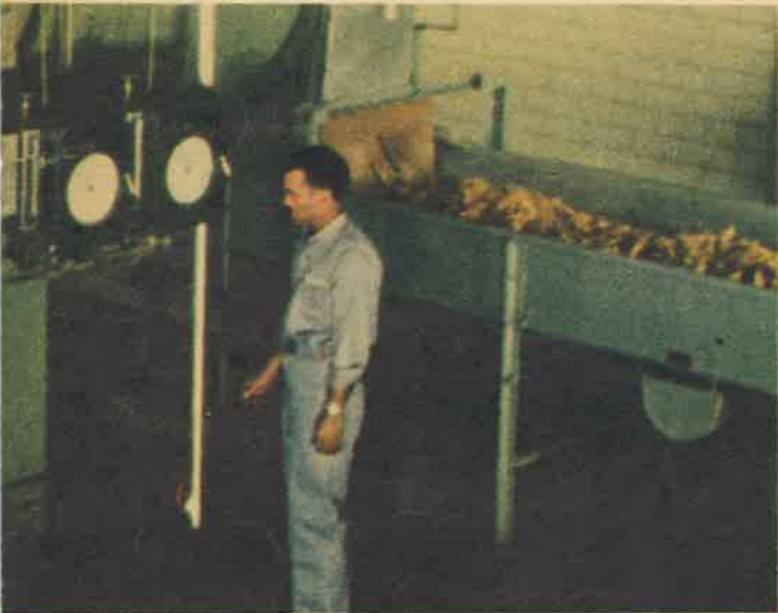
BLENDED and moisturized to Lorillard requirements, tobacco moves from casing drum (above) to cutting, making machines.
