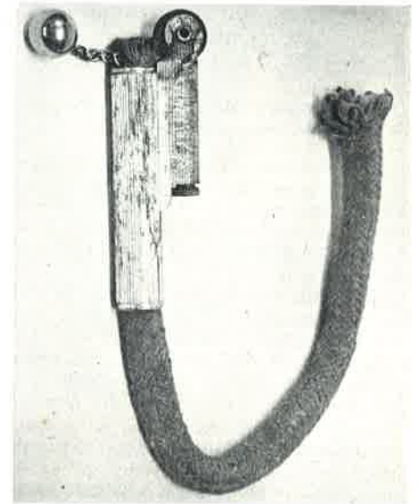
One of the earliest "Kaiser's war" lighters, petrol-less but with tinder wick, cerium flint and wheel, which preceded the petrol lighter
