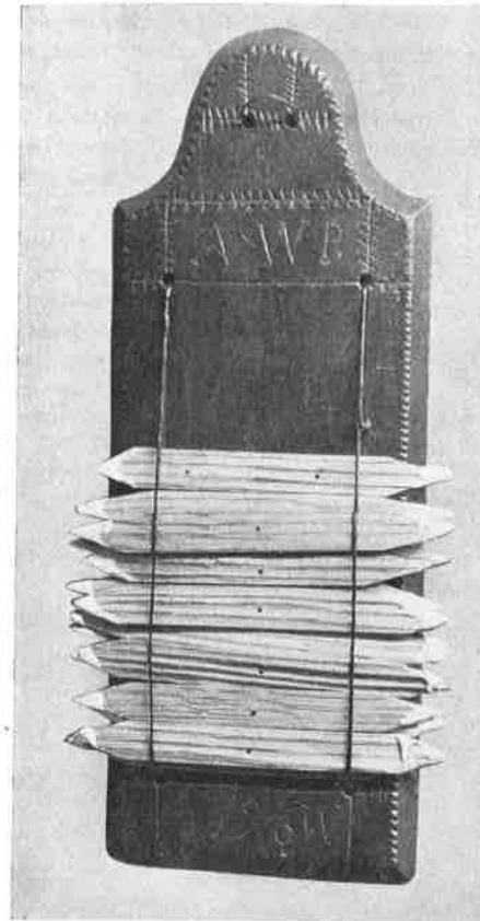
Wood sulphur matches, six inches long, in holder; used in the 16th and 17th centuries and later in conjunction with tinder-boxes. Right: tinder-pistol, a development of the box. Below: tinder-horn for carrying at waist or in pocket
